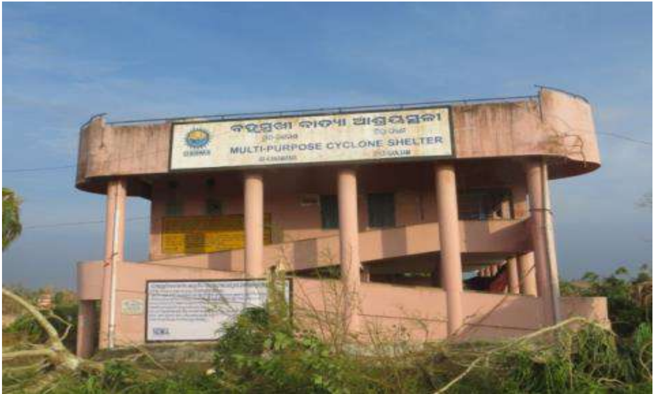
Figure: - 3 Cyclone centres Build by the Govt. of Odisha at Ganjam districts for save of people during cyclone
