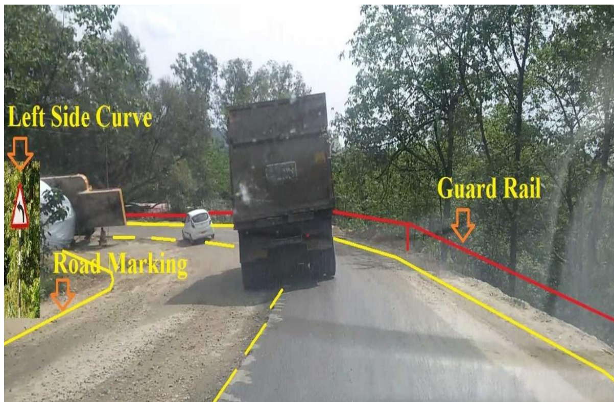
Fig 1.9: Suggestions for improvement for Mubarakpur accident spot. Source: Site visit photography.
