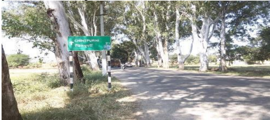
Fig 1.2: National Highway-3 with Sign Board.
