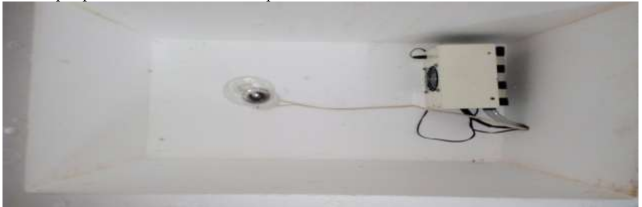
Fig. Cooling unit with test lamp under insulated condition
