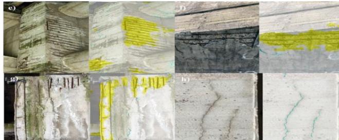
Fig. 12. Test images with high-resolution pier cap(e), abutment(f), pier cap(g), and concrete surface (h).
